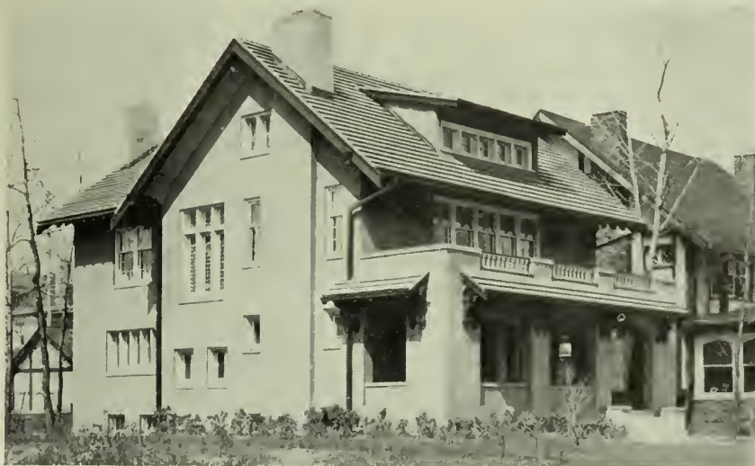
HOUSE AT COLUMBUS, OHIO. Roofed with Ludowici-Celadon Company T-14 tile. Frank L. Packard, Architect.
